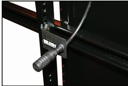
Belden's AEHC system utilizes pressure sensing to dynamically adjust for speed, resulting in perfect balance between intake and exhaust air volume.
